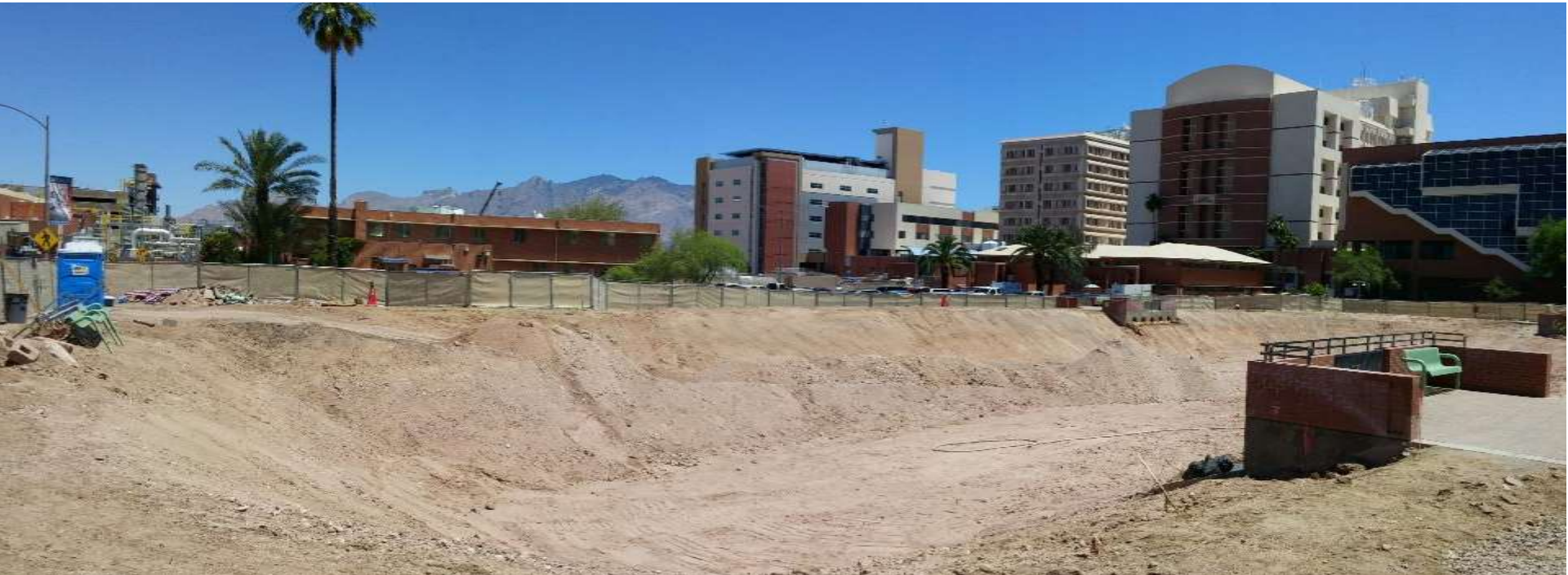
Cherry Avenue detention basin excavation
