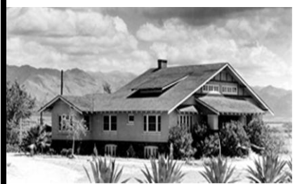
1920 – Lester Built House
